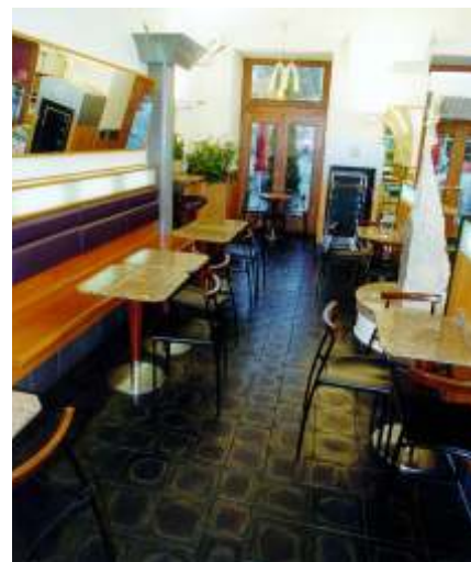
A tile made of cast basalt size 200/200 or 250/250 mm Comes from molten basalt of temperature around 1300°C / 2372°F
