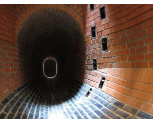
Figure 5 Connection to the “K” interceptor (1200/1800 mm profile)
