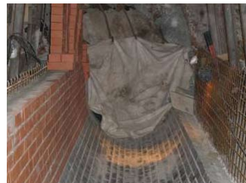
Figure 10 The construction of the connector to the "K" interceptor
