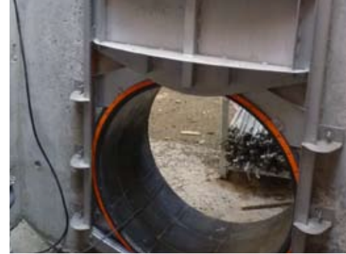
Figure 6 Ring made from calibrated radial-shape cast basalt elements
