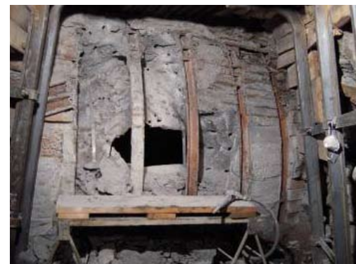
Figure 9 The opening into the "K" interceptor
