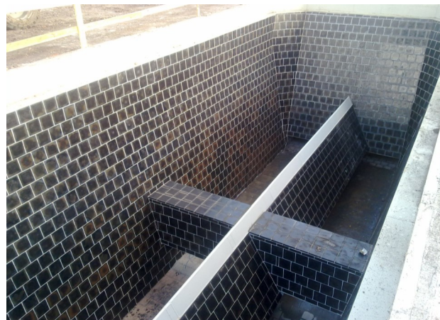
Plain tile as lining of deep coal bunker
